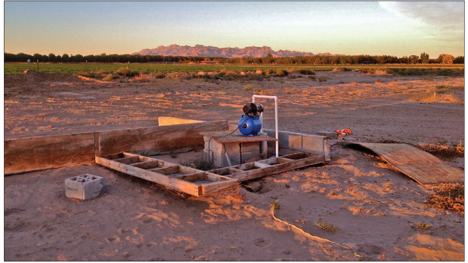
A typical (unsheltered) private wellhead found in colonias in New Mexico.
