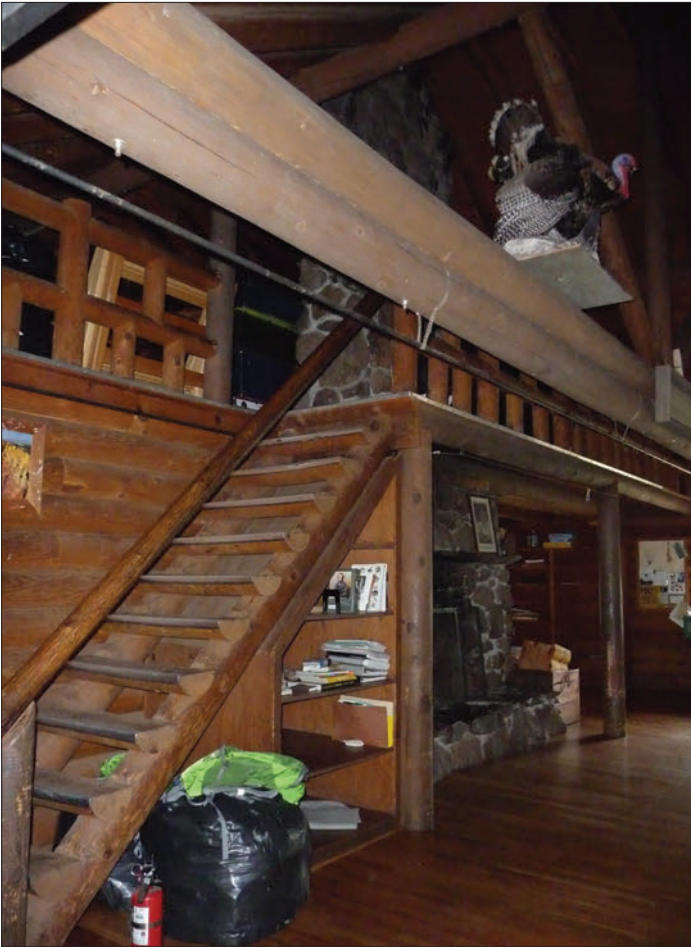
Loft inside cabin.
