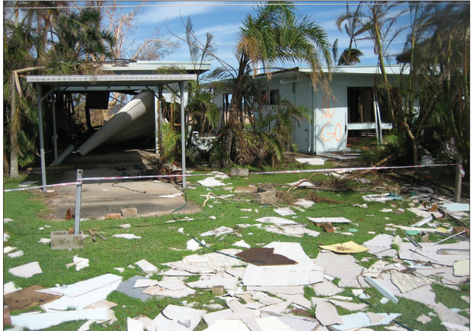
Tully Heads with asbestos-containing material on public and private land.
