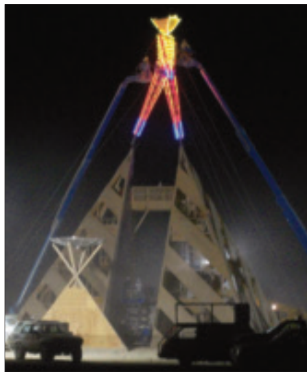
The Burning Man statue, referred to as “the Man,” under construction. A new design for “the Man” is done every year.
